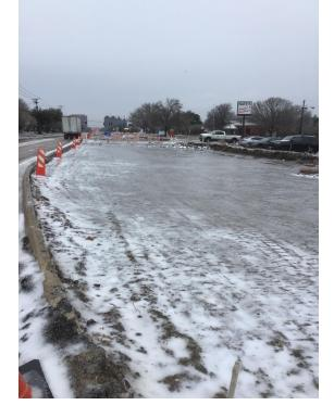
After several weather-related delays, the main lane paving of the Midway Road Revitalization Project from Belt Line Road to Proton Drive is scheduled to begin the week of February 13. Activities will include the fine grading and lime stabilization of the subgrade, installation of the reinforcing steel and joints, and finally the placement of the street pavement.
